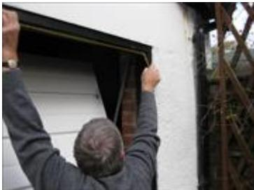
With a tape measure, measure the opening from wooden post to wooden post at the top of the garage door. Do not measure the width of the garage door.
