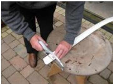
Make a mark with a pencil on the Weather Stop Top Seal where the seal needs to be cut to fit the opening.
