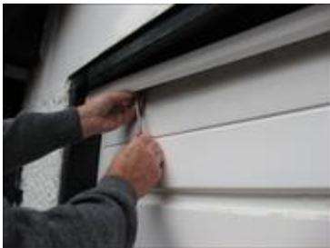
With the garage door half open, position the Garage Door Top Seal where you have marked the frame. Then put the washer over the screw and then put screw through the hole in the top seal and then fix the screw into the head of the frame. Continue this process until the top seal is secured tightly.
