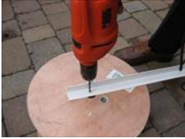
With a pencil make a mark approximately every 300mm. Using a 6mm drill bit, drill holes through the top seal where you have made marks on the top seal. Make sure you remove any excess plastic to make a clean hole.
